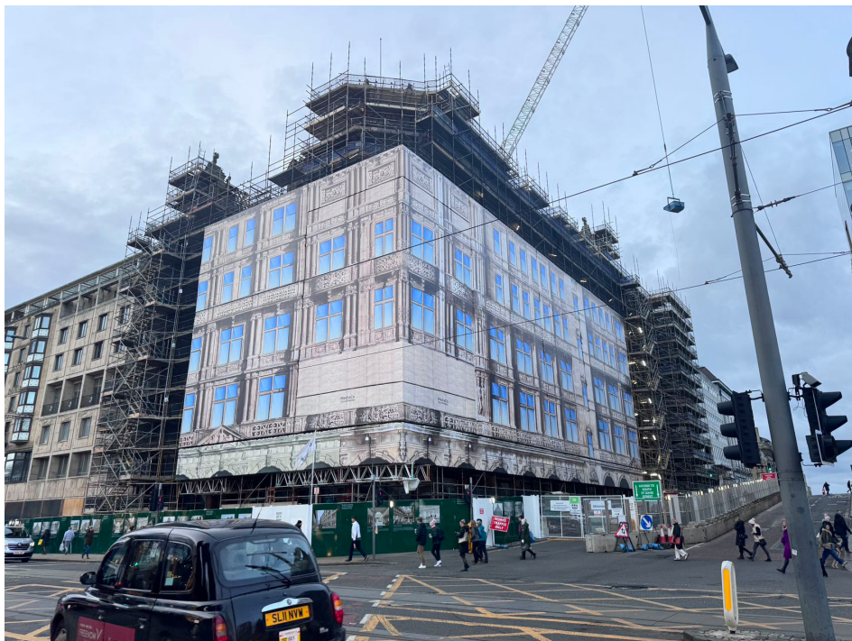
Figure 8, "The Jenners Building undergoing renovation", photo by the author.
