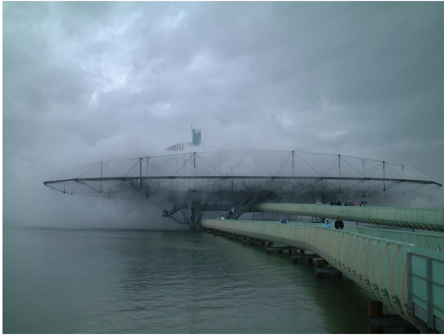
Figure 14. Blur Building enveloped by mechanically produced fog at Swiss Expo 2002, Yverdon-les-Bains, Switzerland. Designed by Diller + Scofidio. Photograph by Norbert Aepli (2002). Source: Wikimedia Commons.
